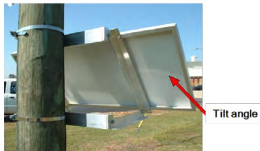
Figure 61 – Mounted Solar Panel
