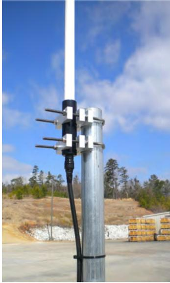
Figure 84 – RF Antenna to Mast
