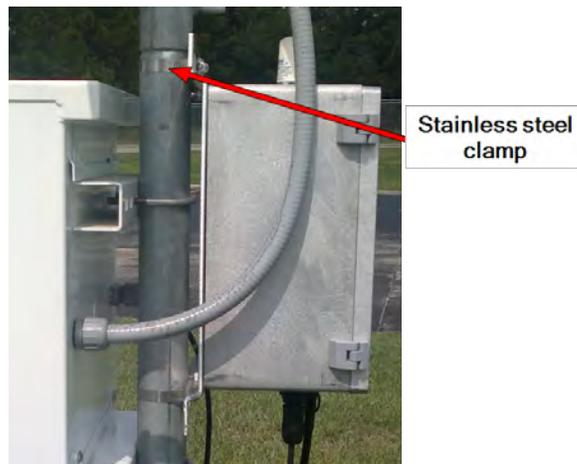
Figure 41 – Positioning the Gateway
