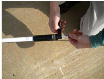
Figure 83 – Weatherizing RF Antenna
