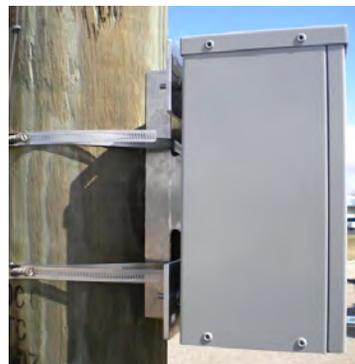
Figure 68 – UPS Attached with Clamps
