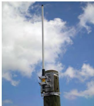
Figure 53 – RF Antenna Bracket
