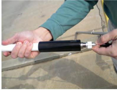
Figure 31 – Attaching the Coaxial Cable
