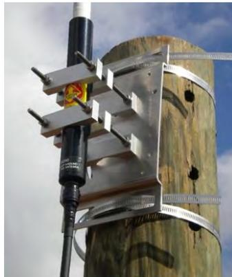
Figure 55 – Weatherized Connection
