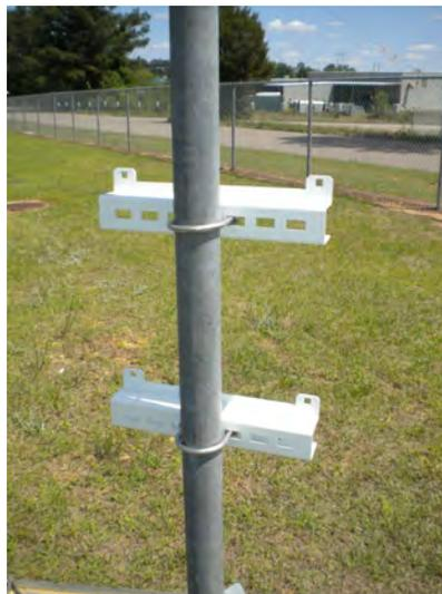
Figure 34 – Installing Pole Brackets
