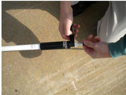
Figure 32 – Weatherizing the RF Antenna
