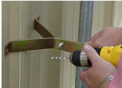
Figure 80 – Lining up Second Pole Bracket
