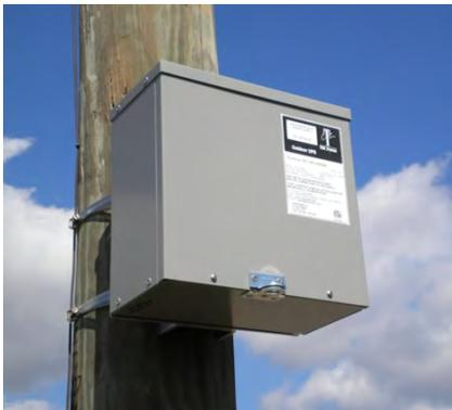
Figure 67 – UPS Attached to a Large Pole
