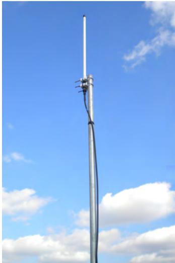
Figure 85 – Securing the Coaxial Cable
