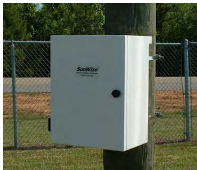
Figure 60 – Mounted Battery Box
