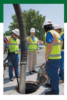
Depending on the slopes of the pipes and the configuration of the manholes, many adjacent segments can be monitored simultaneously with a single sensor. This unique capability allows multi-segment monitoring from a single site, making SmartCover the lowest cost-cost-persegment monitoring system.
