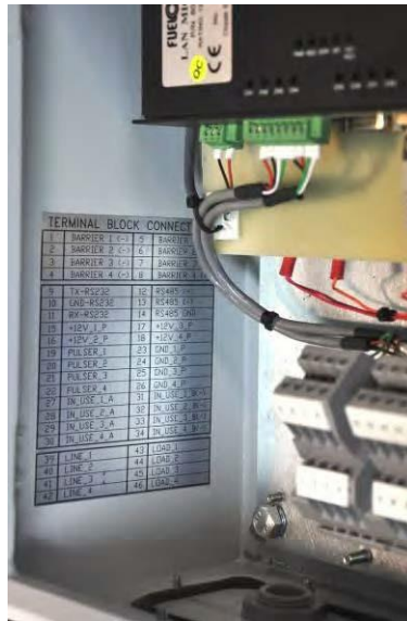
Figure 3-8. Terminal Block – Mechanical Pump - Wiring List Label Installed
