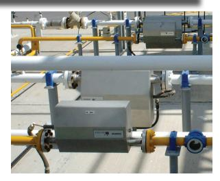
Neptune M-dot Coriolis mass flowmeters measure every fluid and vapor flow.
